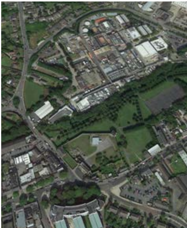
Aerial Photograph, Swords Industrial Area
