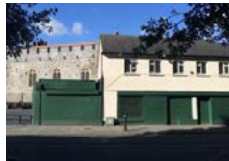
Derelict Buildings on North Street
