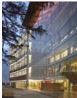
Fingal County Hall
