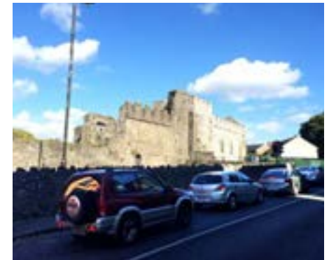
View From Bridge Street - Looking North
