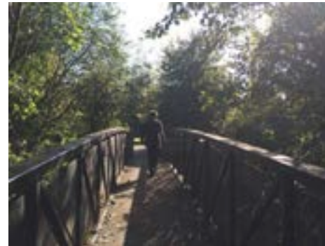
Castle Park - Pedestrian Bridge
