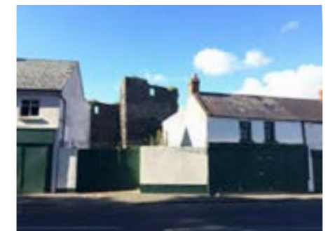
Derelict Buildings on North Street
