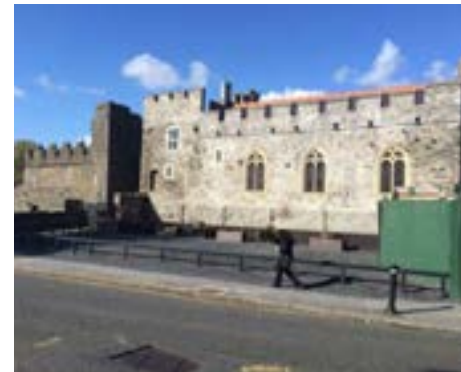
View From Main Street - Looking North
